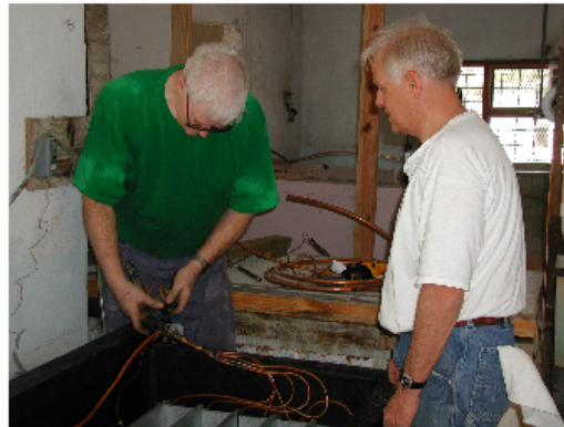
Above: Bob Port and Bob Shelton install refrigeration lines for new machines.
