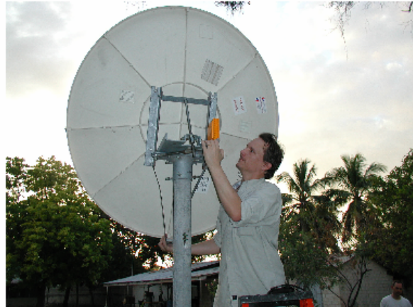
Above: Budd installs new dish.
