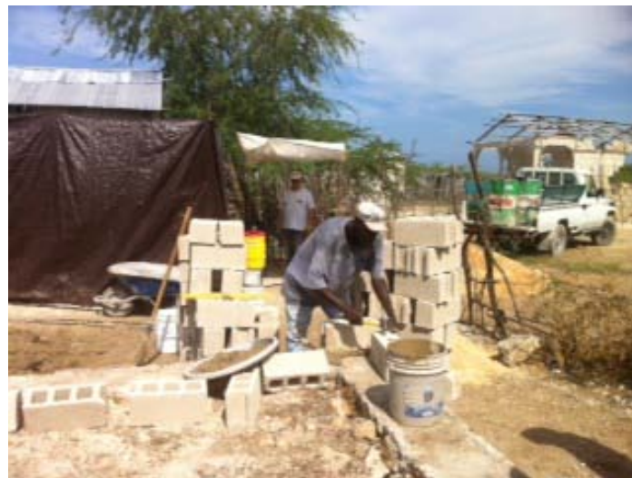
Construction begun, old house in the background.
