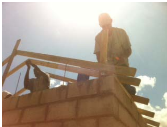
House almost finished
