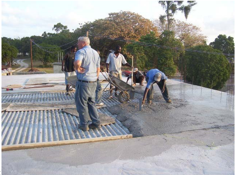
Second Story Floor.jpg
