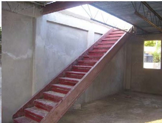
Metal stairs to the second floor
