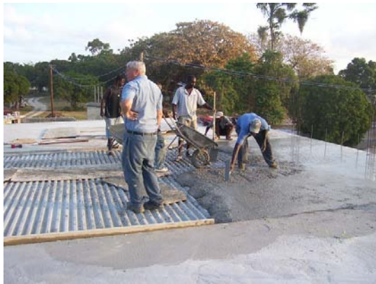
A team pours the second floor
