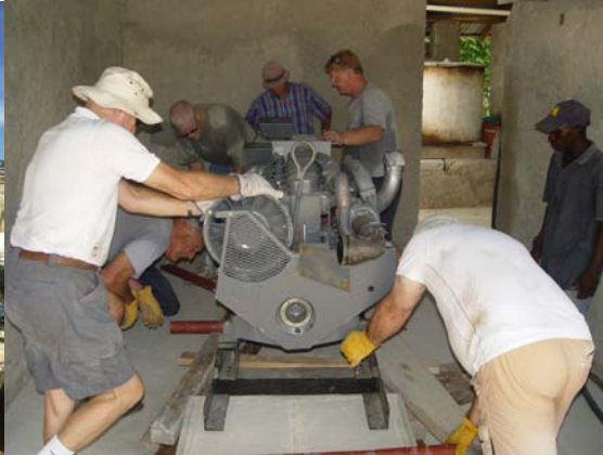
Installing a generator
