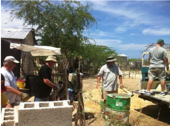
Laying block for the walls of a house
