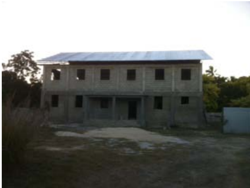
New roof on the library/resource center
